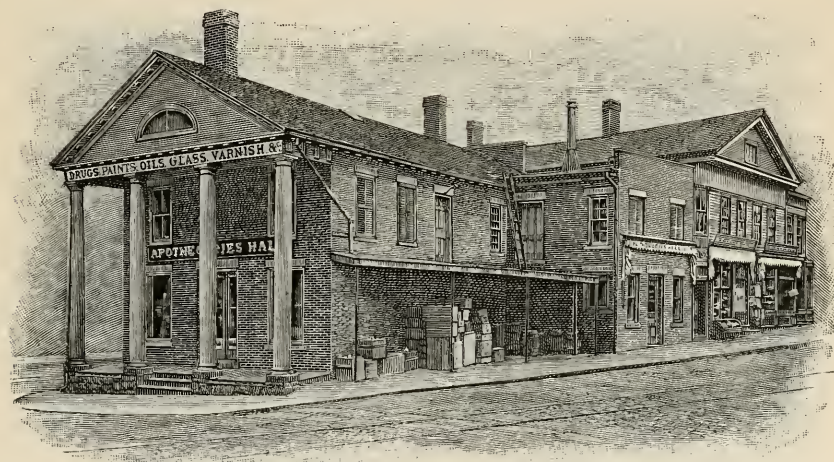
STORE OF THE APOTHECARIES' HALL COMPANY, AT THE JUNCTION OF BANK AND SOUTH MAIN STREETS, FROM 1849 TO 1891.†
